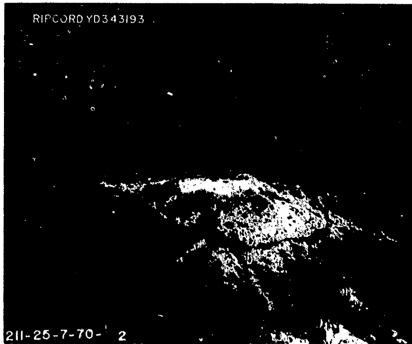
FSB Ripcord abandoned, July 1970
