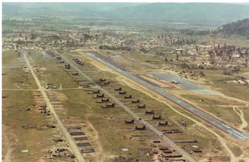
Heliport and airstrip, Camp Radcliff
