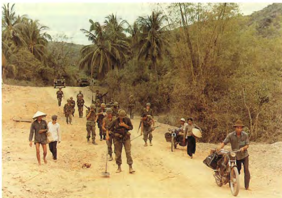
Engineers clear a stretch of Highway 1 in Binh Dinh Province.
