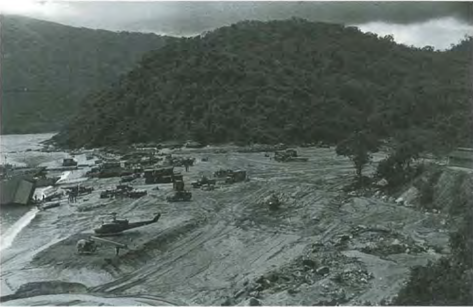
The port under construction at Vung Ro Bay
