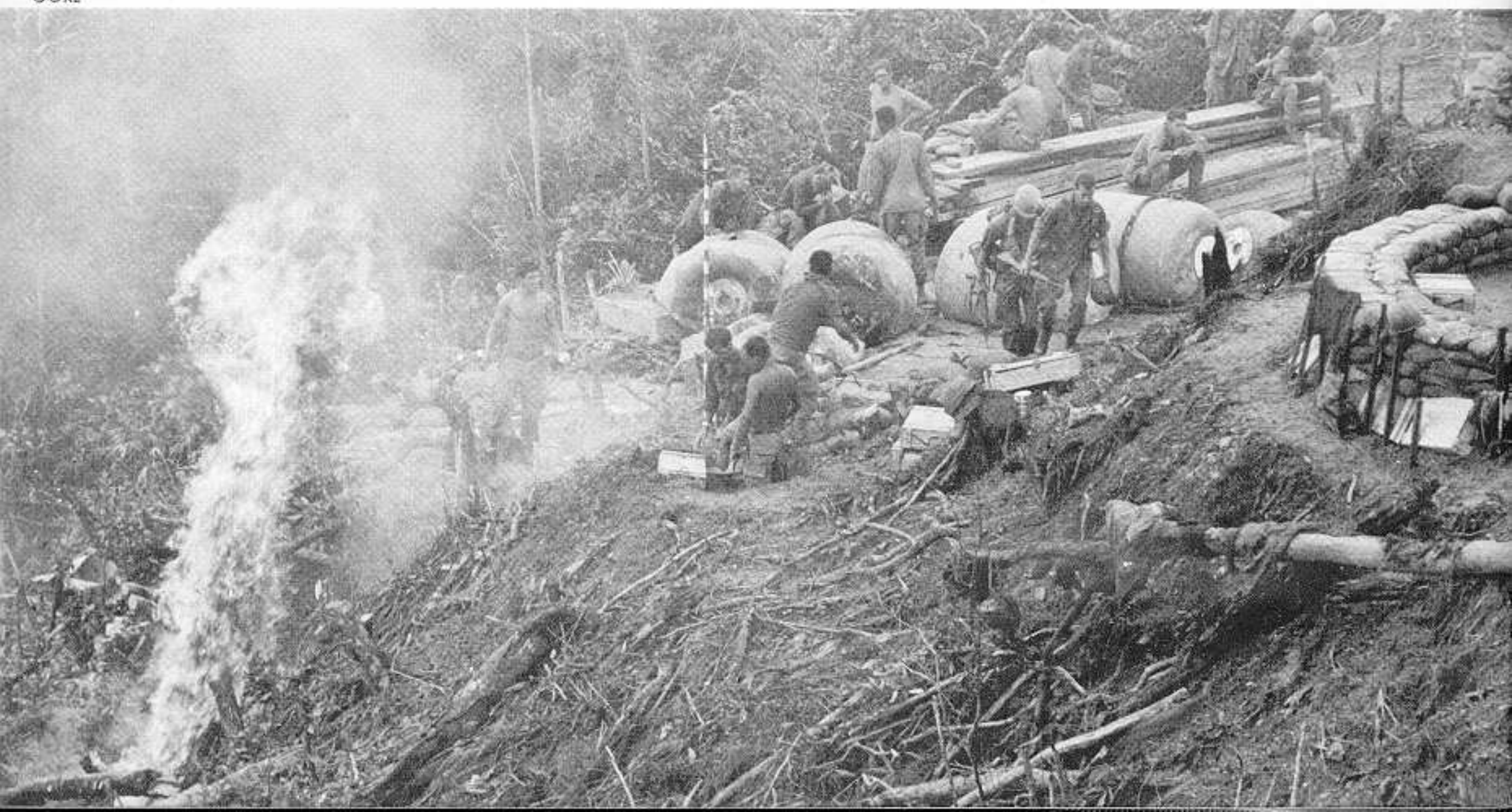
As Fire Base Sledge takes shape, Screaming Eagles clear the surrounding brush.
