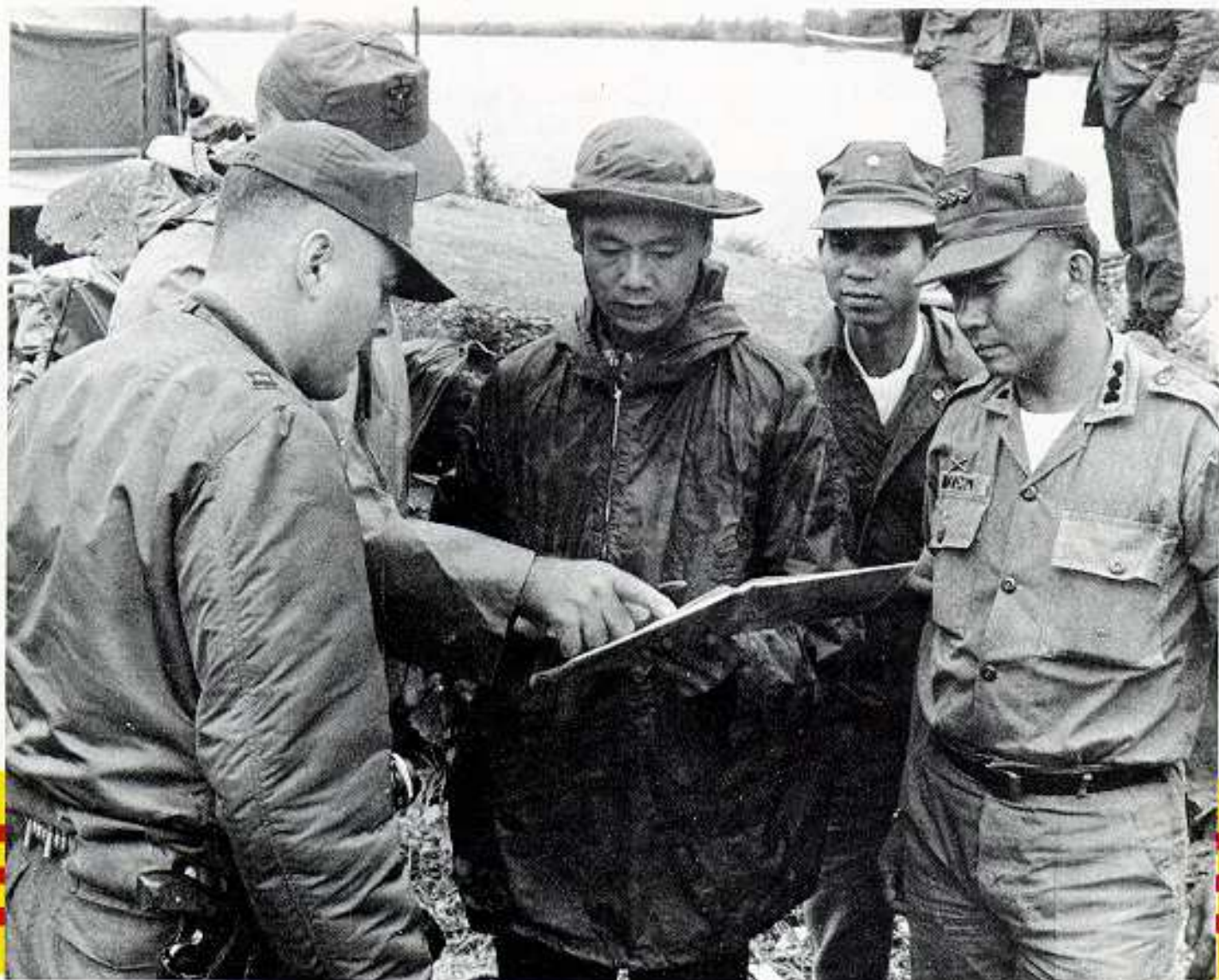
Col. Chism (background) and Col. Than examine plans for another building project in Huong Dien District as Dai-uy Bien, the district chief looks on.
