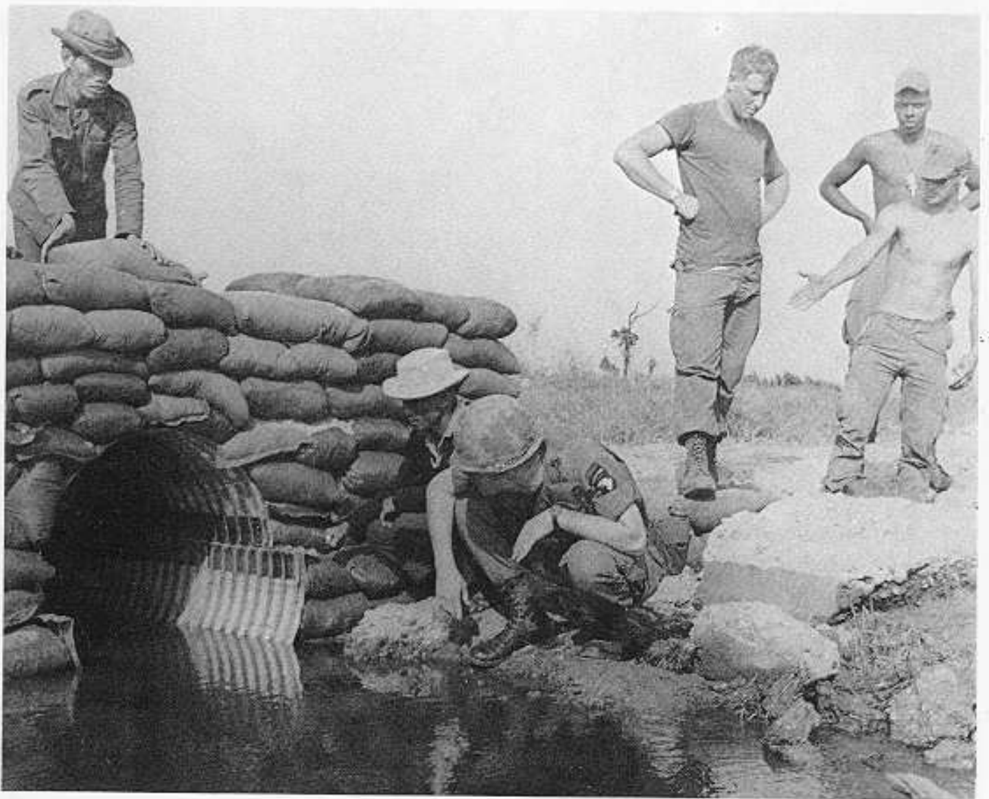
Screaming Eagles from the 326 Engr. Bn. (Ambl.) examine a recently completed culvert along the Street Without Joy.
