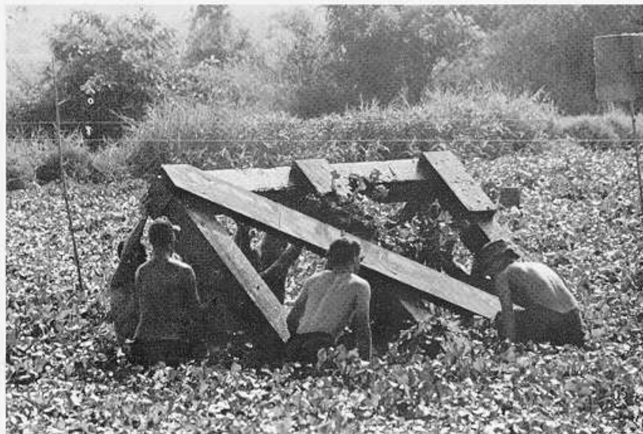
Waist-deep in water, engineers prepare to place a bridge section.
